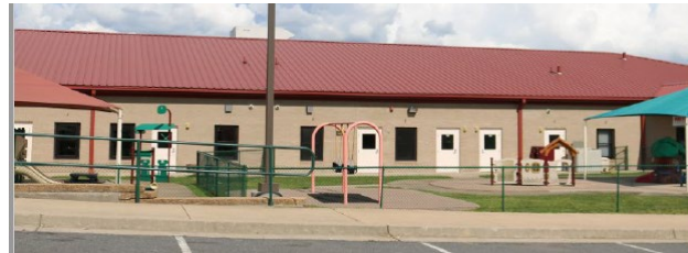
Child Development Center, Building 3349 7687 Georgia Avenue Facility Director: Valerie Hammond Total Employees Assigned: 33 Services: Full Day Care - Infant to Pre-school Pre-COVID Spaces: 102 Post-COVID Spaces: 76
